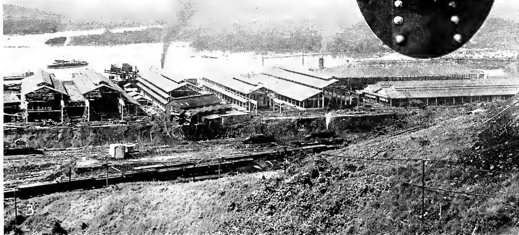
1. Rear Admiral Harry Harwood Rousseau, builder of the canal terminals. 2. Sinking concrete caissons for the foundations of the terminals. 3. Pacific terminals, with a glimpse of the canal in background.
