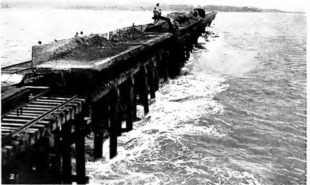
1. Breakwater at Naos Island, on the Pacific side, looking back toward the land, with Panama city in the right background. 2. Toro Point Breakwater, at the Atlantic entrance, showing stone being dumped from a Lidgerwood train.
